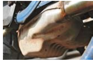
The collector box is prone to rot.
