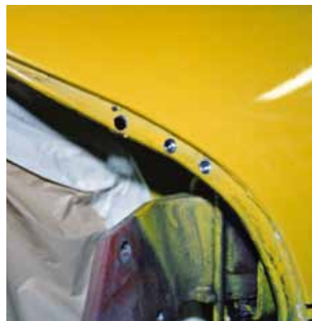
4-1c. Drill out weld on door edge ...
