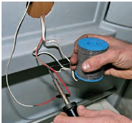
Picture 9. This step must be done by a qualified electrician. A large hole cut in the shower trim allowed access to the cables. The fan positive terminal was given a permanent (fused) connection.
