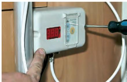
Picture 8. Graham fixed the control box in place. Luckily, he found a fused 12V feed from inside the wardrobe base (otherwise, he would have run a new one from the battery).
