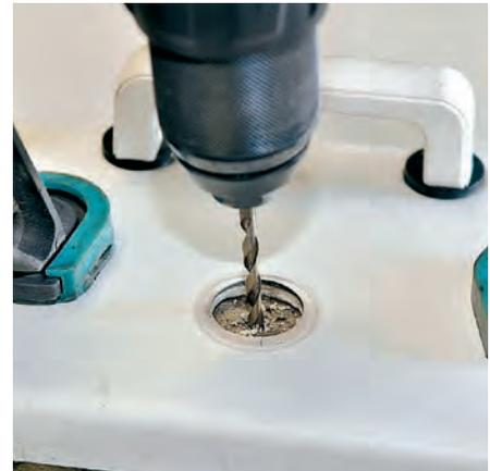
Picture 4. ... and a strong piece of scrap wood tightly clamped to the back, before carefully and accurately drilling a pilot hole, right in the middle of the hole for the old lock.
