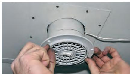
Picture 8. A smaller ceiling plate was fitted, and finished off with the Dometic trim plate. The stainless steel screws we used came from Screwfix Direct – quite inexpensive.
