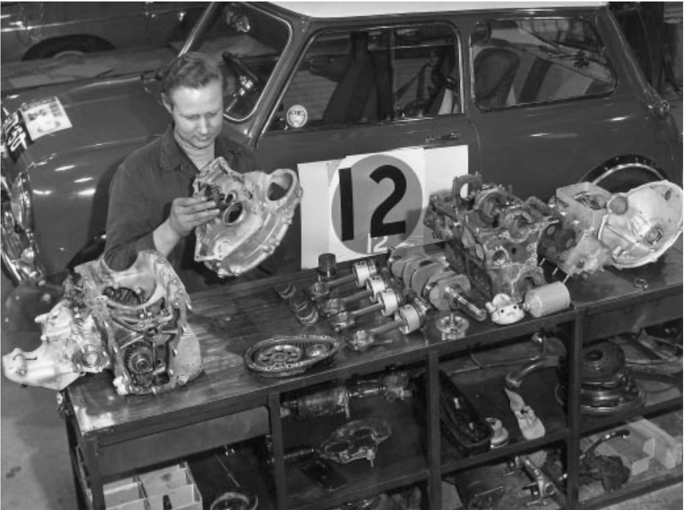
Engine tuning ace Cliff Humphreys assembling a Mini engine.
