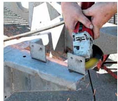
Picture 3. Dave used the angle grinder to cut through most – though not all – of the welds holding each bracket in place.
